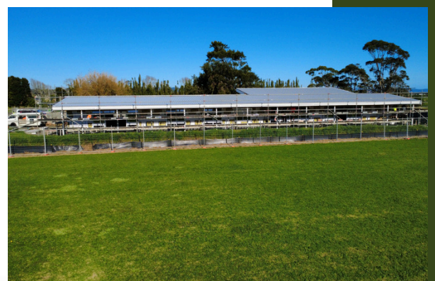
Blomfield Satellite School Construction
