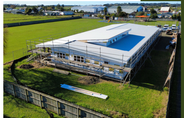
Blomfield Satellite School Construction
